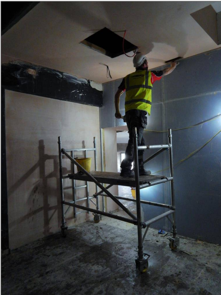
First fix electrics are mostly complete and work has started on lining out the new ceilings and plastering
