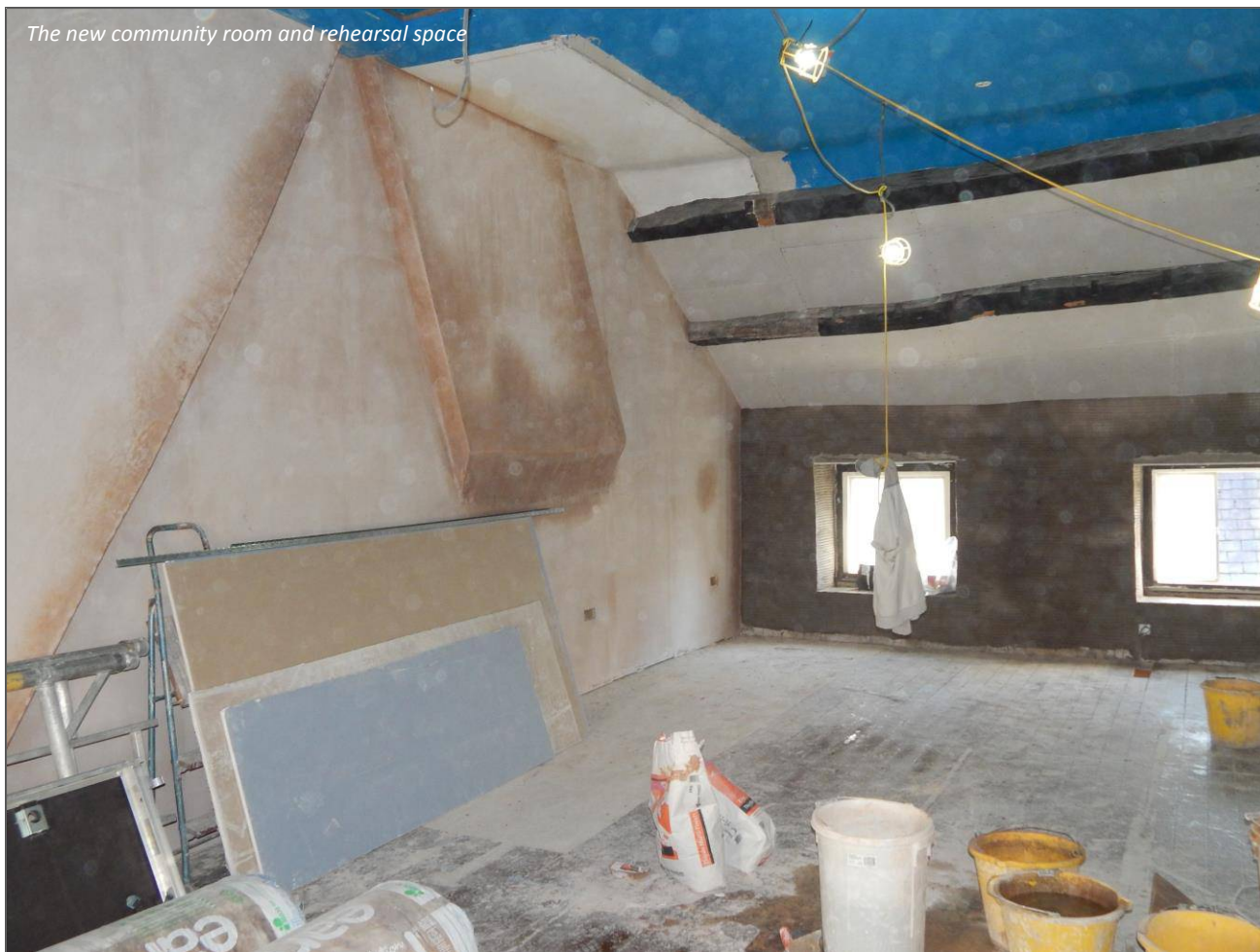
The new wardrobe accommodation on the top floor of 30 Wilson Street – new ceiling lined out, scratch coat to wall and structural roof timbers replaced
