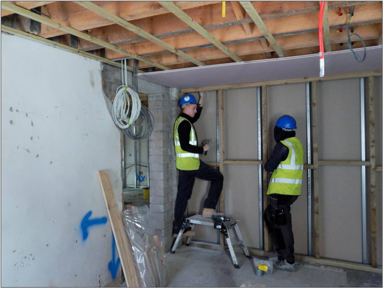
First fix electrics are mostly complete and work has started on lining out the new ceilings and plastering
